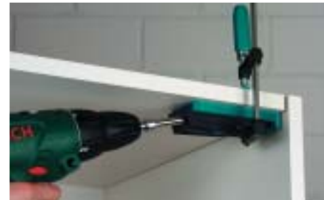
For repairing without removing beforehand
